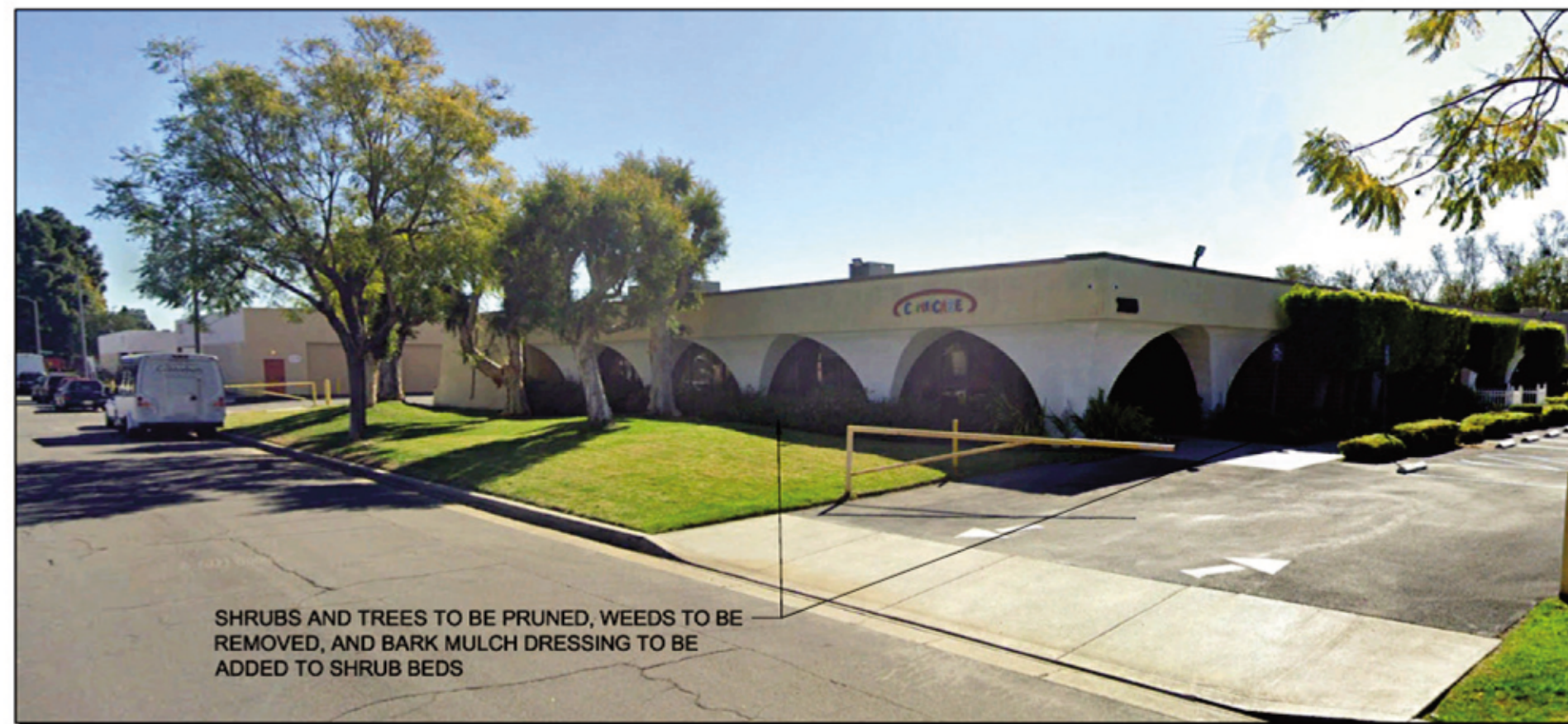
P2 - E. Dominguez Street - View of North Building
