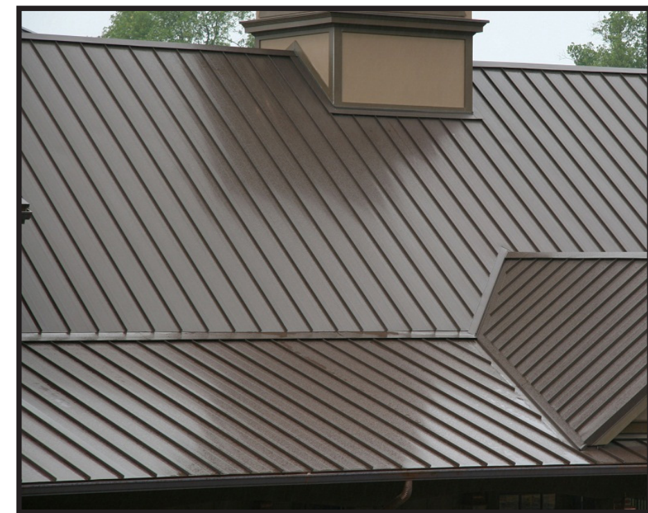
05 STANDING SEAM METAL ROOF COLOR: DARK BRONZE
