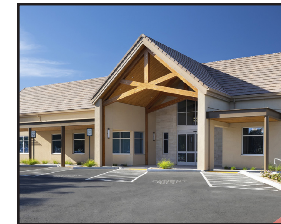
09 EXPOSED WOOD TRUSS
